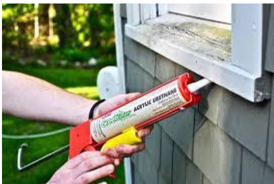
Air Sealing Exterior Joints
