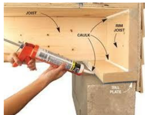
Air Sealing Interior Joints
