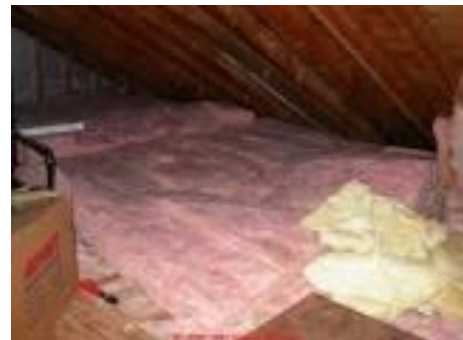
Renewed Attic Floor Insulation
